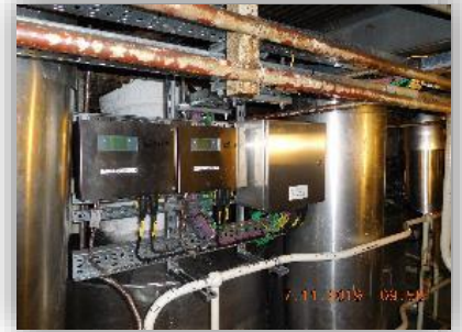
U/S Flow metering
